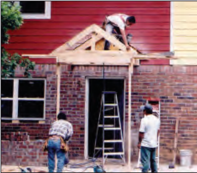
In Georgia, restoring a duplex in Gwinnett County.
