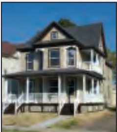
Before, during and after in Syracuse.
